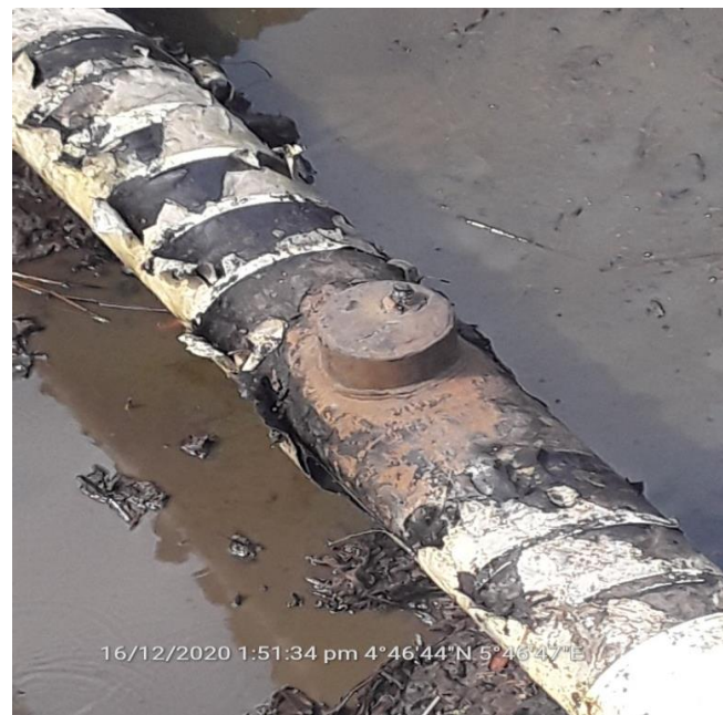
Fig D: Incident Facility during repair
